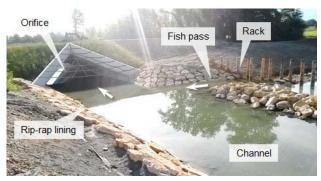
Figure 13: Structures constructed on the Aire River as defined on the physical hydraulic model. A hexagonal orifice and a riprap channel bank lining were adopted upstream from the latter.
